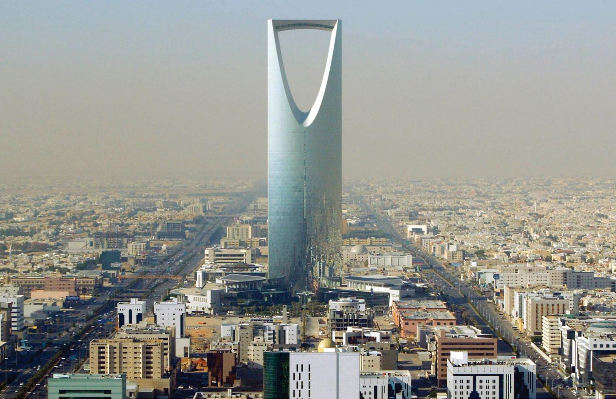
King Abdullah Financial District (Riyadh - KSA)
