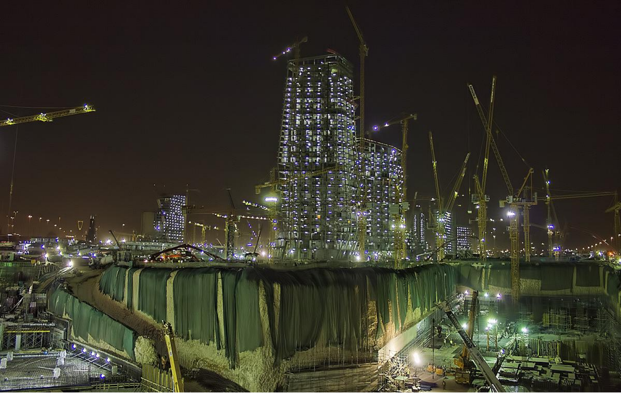
King Abdullah Financial District (Riyadh - KSA)
